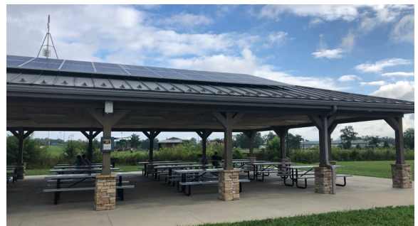
Mills River Park Shelter
