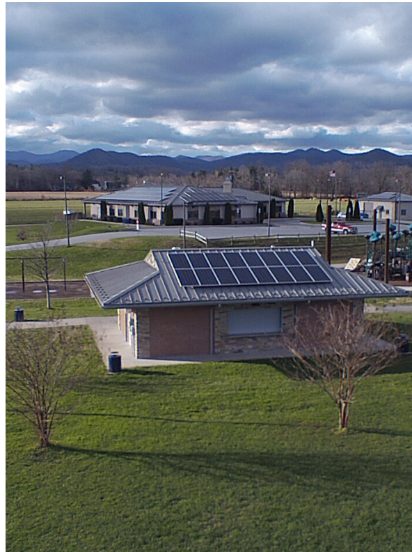
Mills River Park Solar Panels
